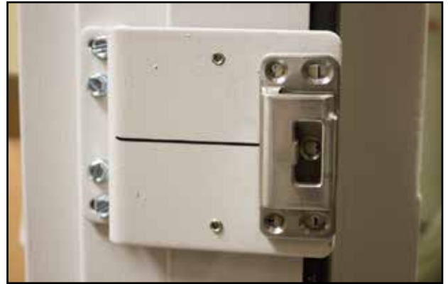
Step 2 - Temporary mount strike to door frame 43" from the floor per LKM10K Lock Series Installation Instructions
