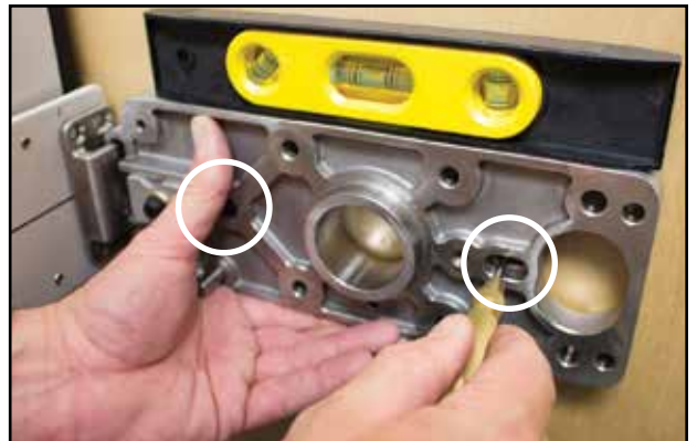
Step 3 - Align the Bolt Position Fixture on the door without touching the strike.
