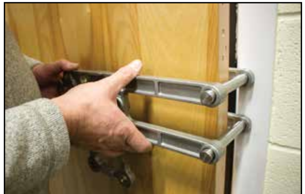
Step 9 - Slide the Front Plate Fixture over the alignment rods.
